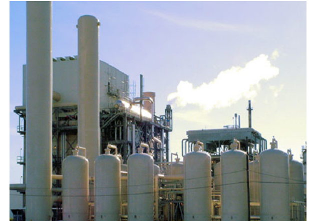
Linde, Texas, STR, HT-shift, PSA NG, 110000 m 3 /h, 99.99% pure H 2
