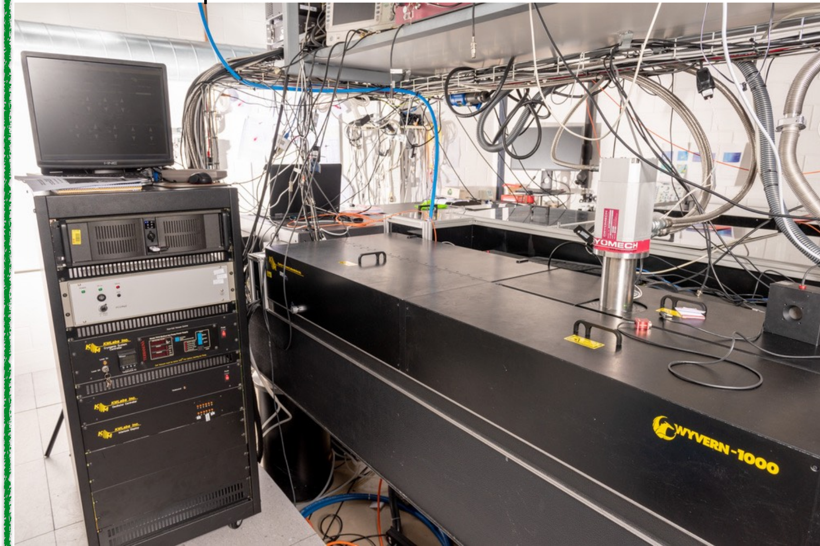
Complete beam enclosure
