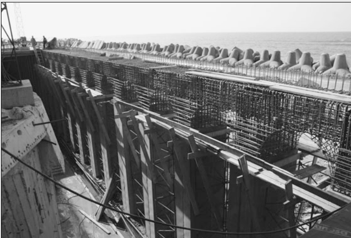
Reconstruction, using high-performance stainless steel reinforced concrete, of the 100 external combs supporting the peripheral slabs. The columns are called 'combs' because they have a wave-breaking effect. In the background you can see the sea and temporary dyke that was built to keep the construction site dry, as well as the tetrapods maintaining the dyke. (© Christine RAYNAUD - BTPM).
