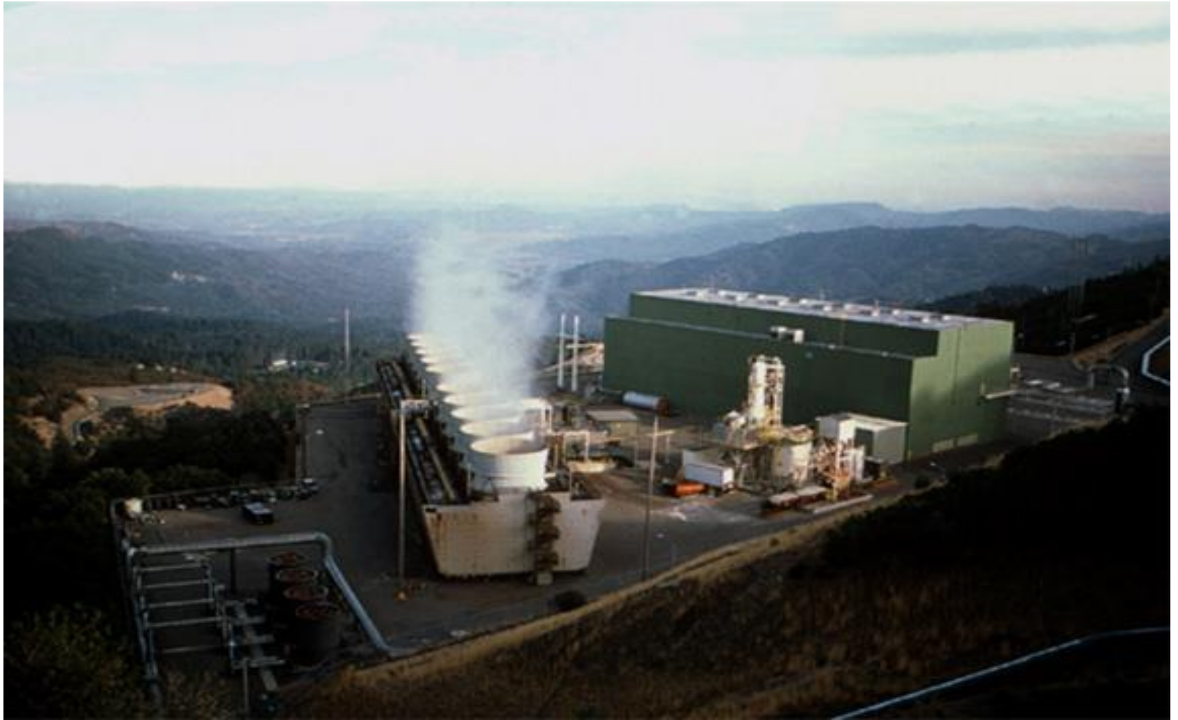
The Geysers dry steam field, northern California, the 1 st USA geothermal power plant (1962) and still the world's largest (1 GW el average).
