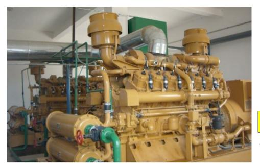
500 kW<sub>el</sub> biogas engine
