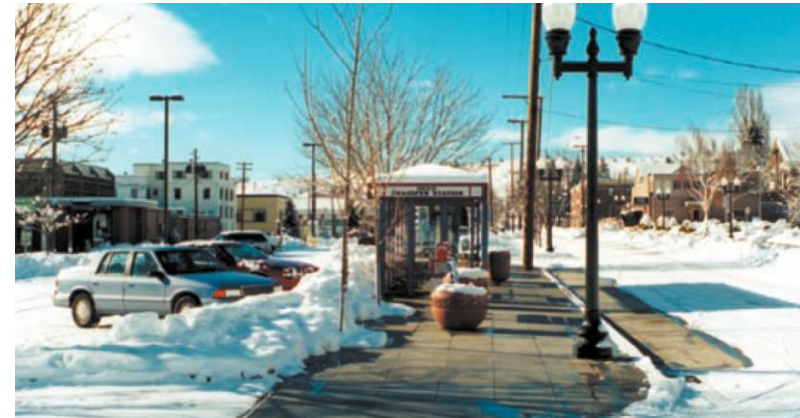
Klamath Falls, Oregon, a geothermal district-heating system keeps the sidewalks clear and dry at the Basin Transit station after a snowfall
