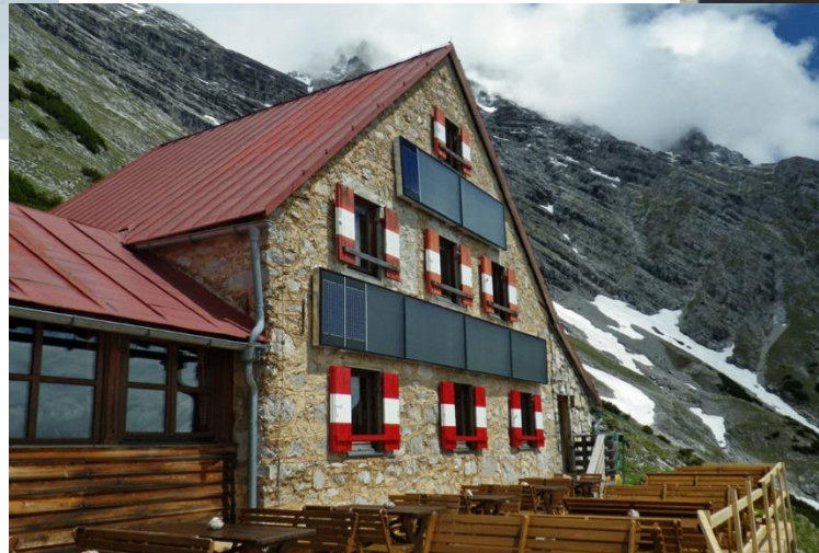
12m 2 air collectors for Bettelwürfhütte, Austria (source: Grammer Solar)
