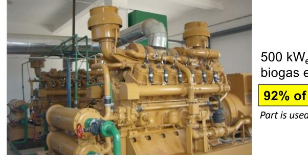
500 kW<sub>el</sub> biogas engine
