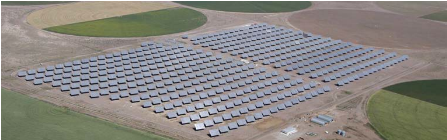
30 MW plant in Alamosa, Colorado, USA (© Amonix)
