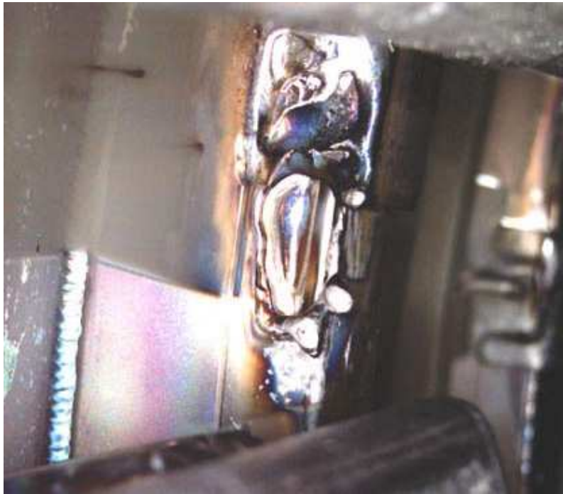
Figure 5: Melting damage to the upper inner wall of JET, thought to be caused by run-away electrons.
