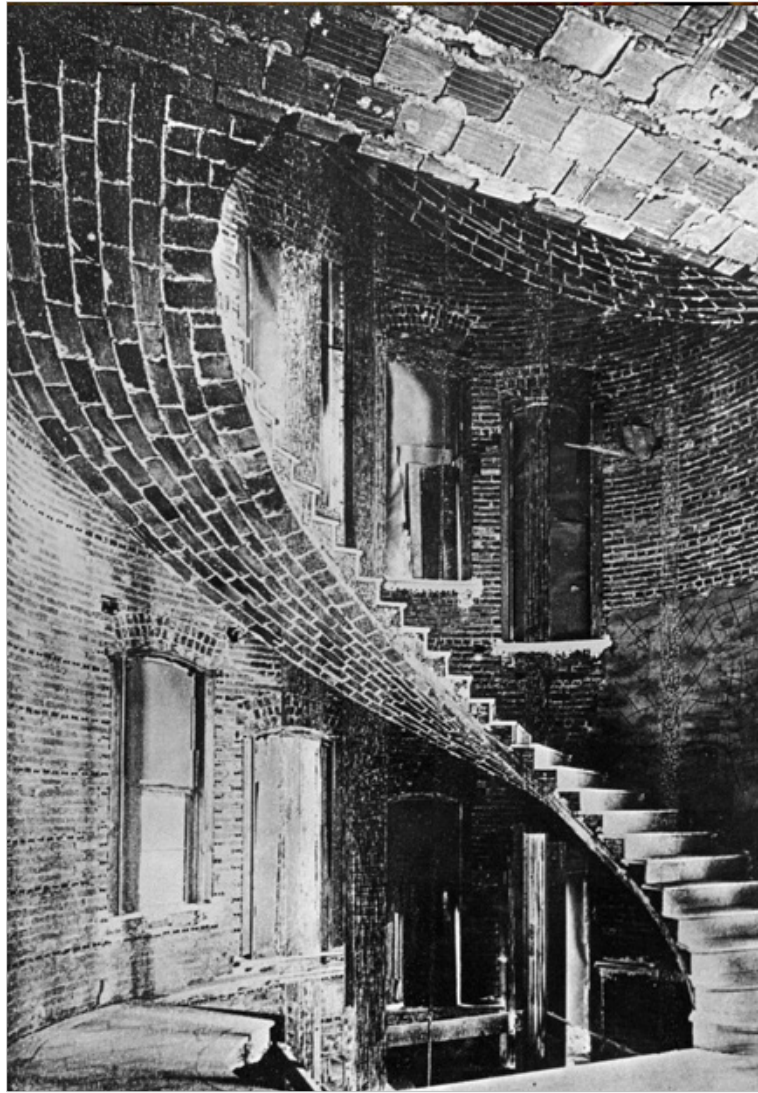
First National Bank – Guastavino 1890
