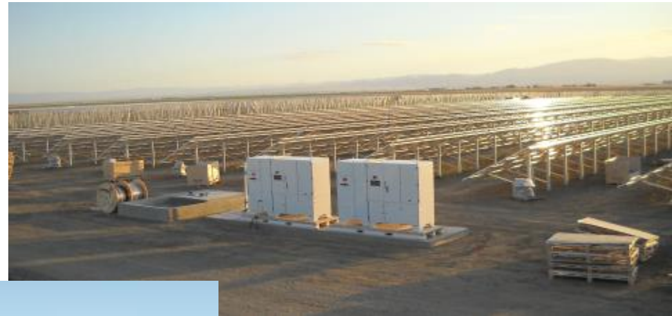
Solaron PV inverters, 500 kW, installed at a 35 MW PV plant, near Coalinga, CA
