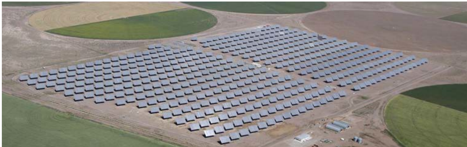
30 MW plant in Alamosa, Colorado, USA (© Amonix)
